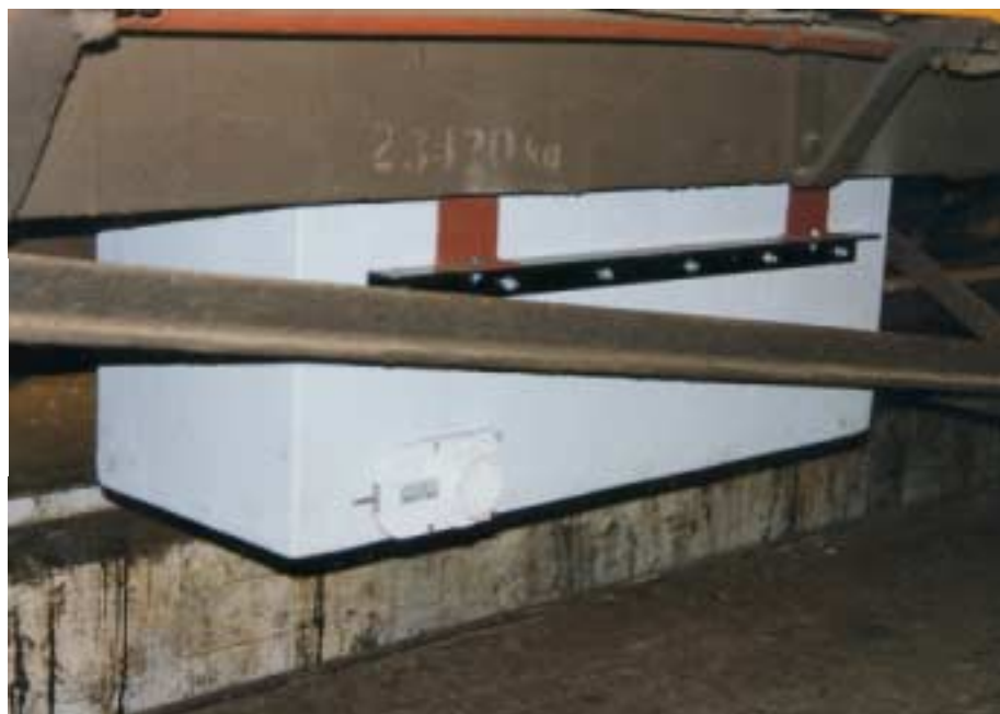
Typical tank installation under a carriage. (The colour does match the rest of the underframe after a time.)
